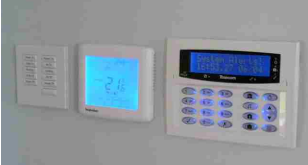
Lutron switch Heatmiser room-stat Alarm panel
